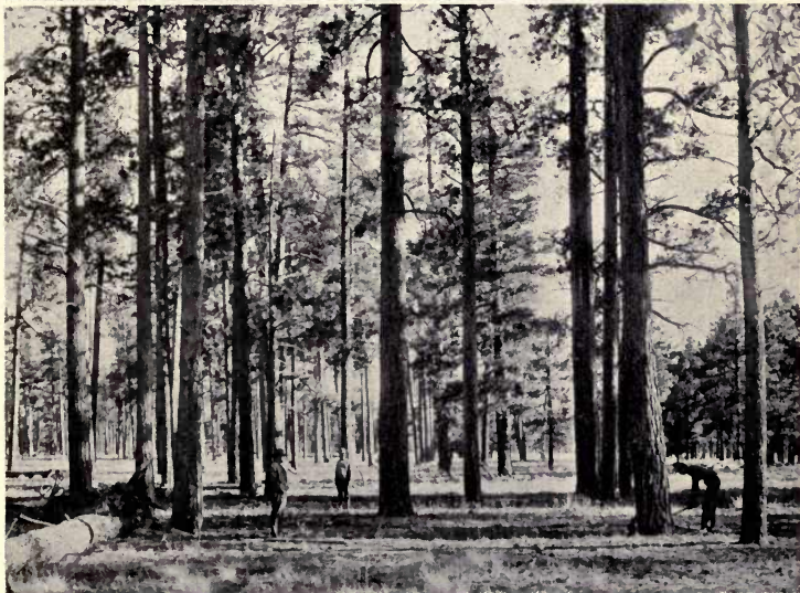
Figure 66. Scene in Montana. Forest officers constructing a telephone line through the Flathead National Forest.
